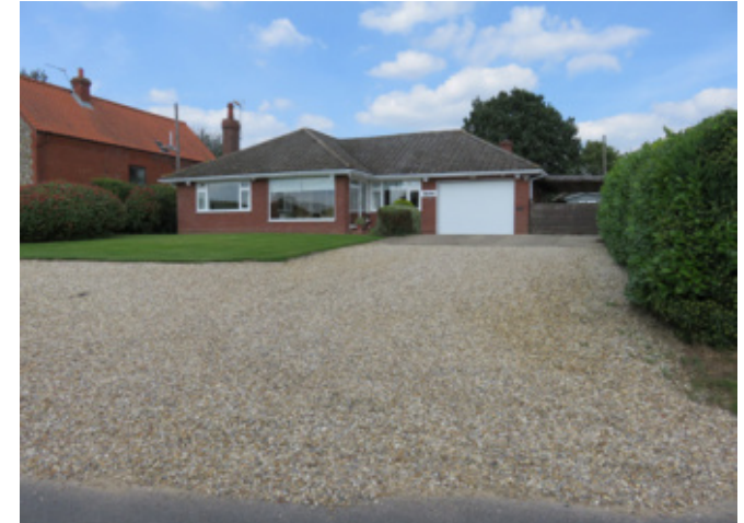
Bungalow on the east-west stretch of Pecks Lane
