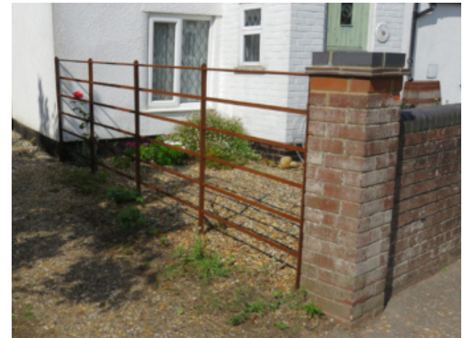
Historic metal railings
