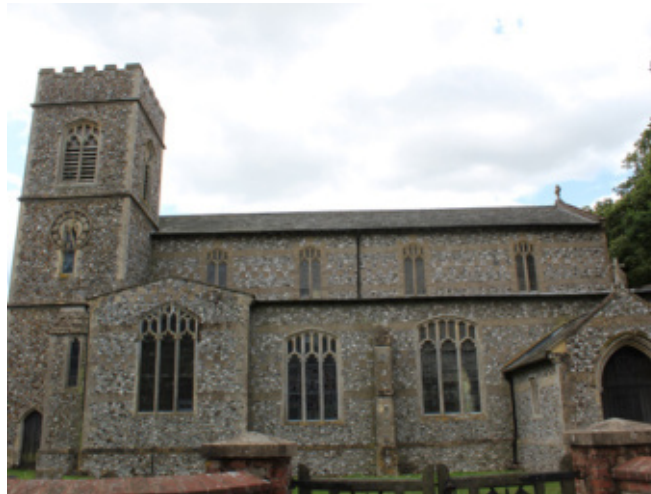
North elevation of the church
