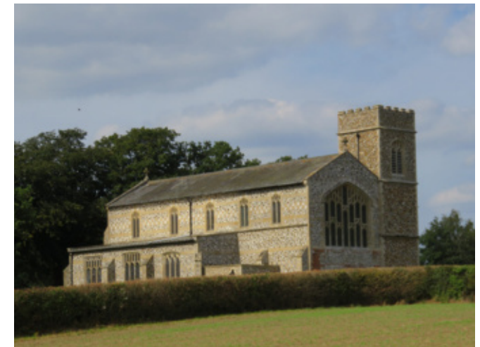
South and east elevations
