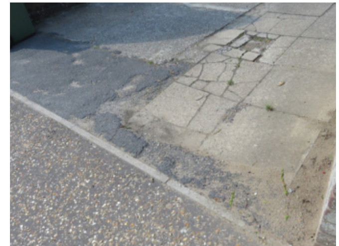
Cracked paving slabs on driveways
