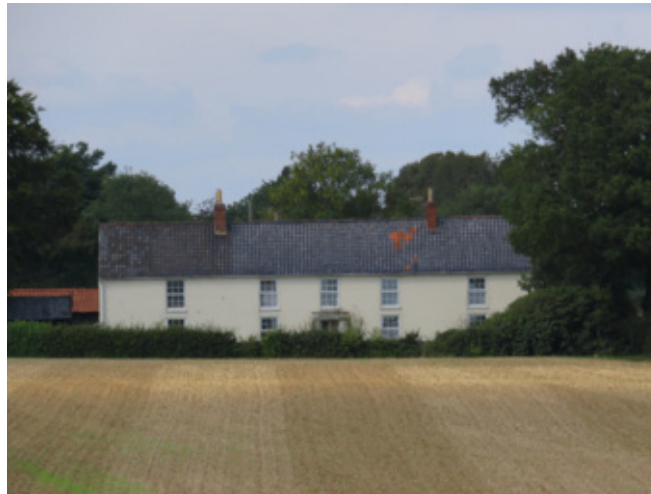
Front elevation of Manor Farmhouse
