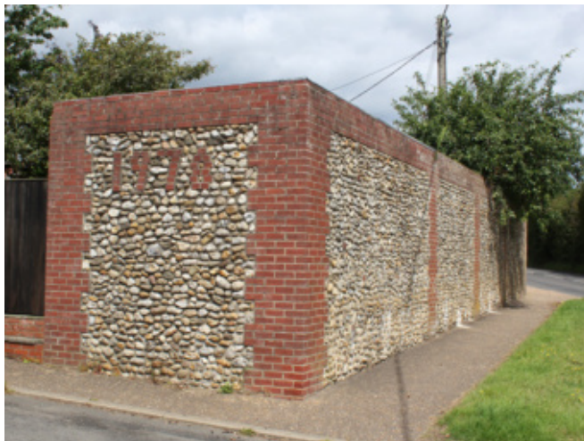
Modern cobble flint and red brick wall with decorative date stone in red bricks
