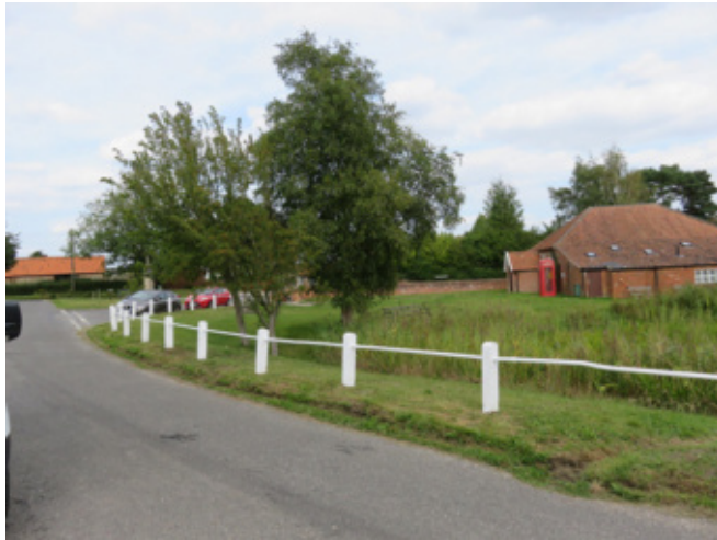
Concrete post and metal rod fencing fronting the pond area of the village Green
