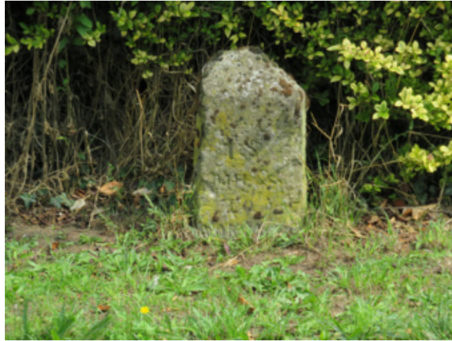
Moss and algae growth on the milestone
