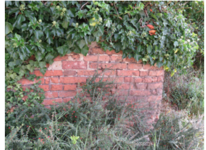
Vegetation growth on brick wall
