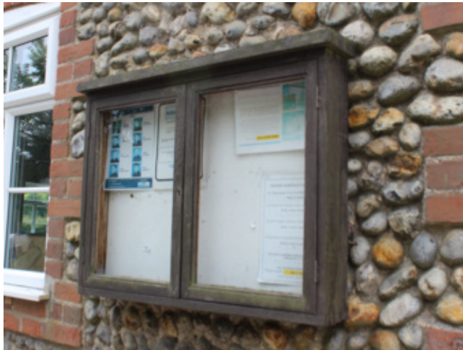
Timber noticeboard located on the Village Hall
