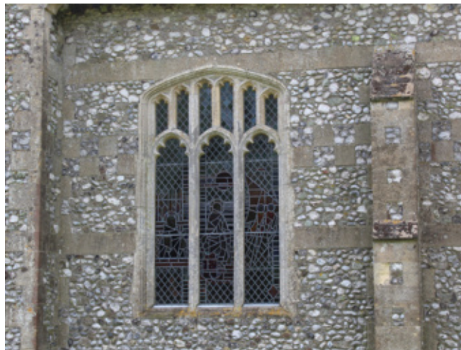
Perpendicular tracery window with stained glass
