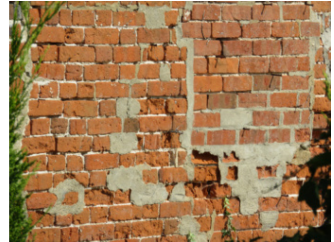
Eroded historic bricks due to cementitious pointing
