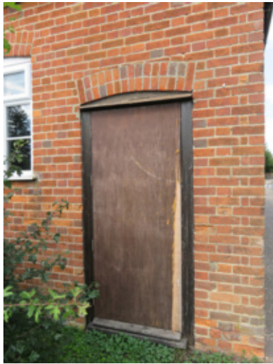
Village Hall rear door
