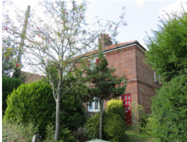
Semi-detached local authority house on Holt Road
