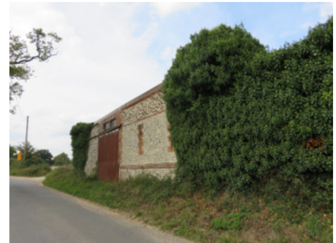
Barn at Merrisons
