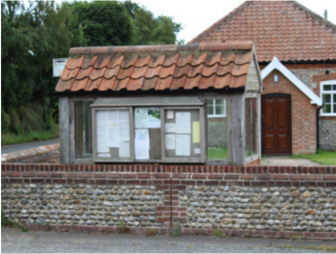
Edgefield bus shelter in front of the village hall
