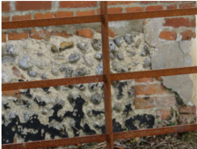
Inappropriate concrete repair
